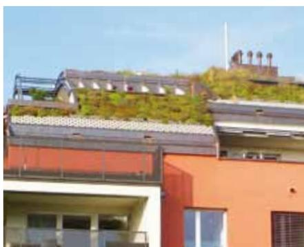
There is no standard solution for barrel roofs. However, solutions specific to your building can be worked out in conjunction with the ZinCo Technical Department, as seen with the roofs of apartment blocks in Pfäffikon in Switzerland (photo above). As gravel edge strips cannot be used for roofs with an extreme pitch, grass pavers ensure a solid and location-stable option for eaves drainage.
