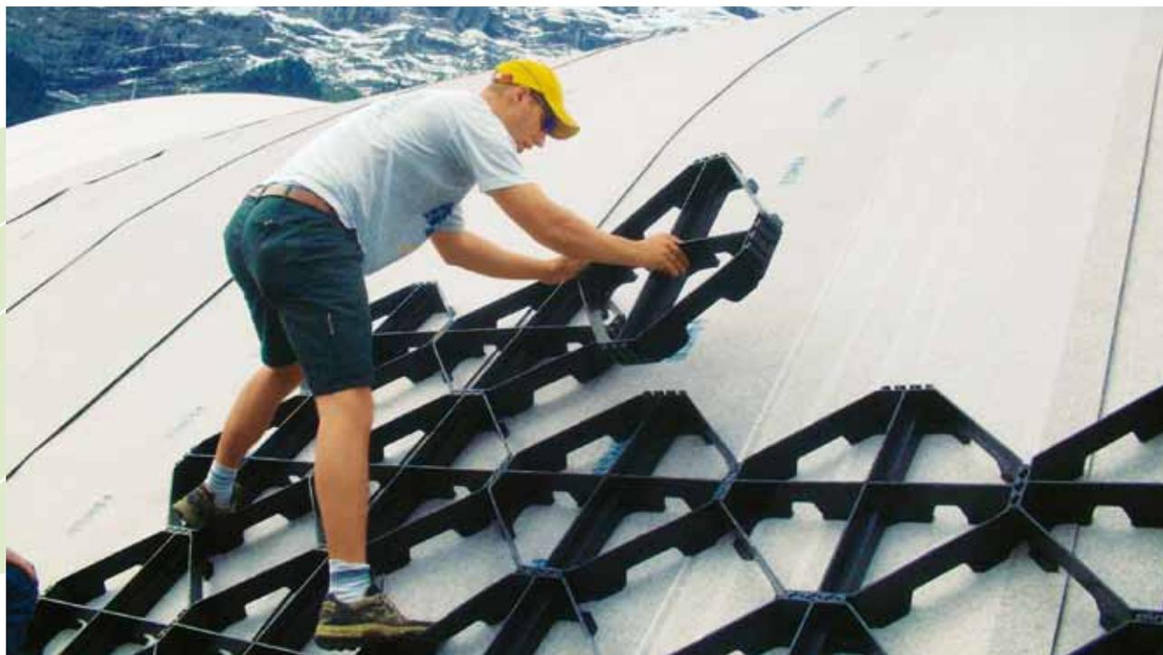
The System Build-up “Steep Pitched Green Roof” based on the ZinCo Georaster® system, as presented here, is suitable for greening roof areas with a pitch of over 25°. The Georaster® elements are 540 x 540 mm in size, 100 mm high and made of recycled polyethylene (HDPE). No tools are required to attach them to each other. The result is a stable and continuous unit.
