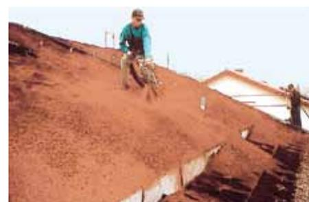
The system substrate “Heather with Lavender-light” is, e.g. delivered in a silo tanker. It is then blown onto the roof using a hose until the Georaster® elements are filled and covered up to about 10 mm over their upper edge.
