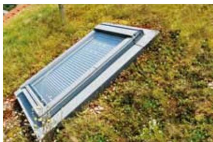
In the case of roof penetrations it is important to ensure that the waterproofing layer is drawn up to at least 100 mm above the upper edge of the substrate layer. Green roof build-ups can be bordered using the stainless steel Eaves Profile TRP 140 in combination with shear retainers (either Support Bracket TSH or Shear-Fix LF).
