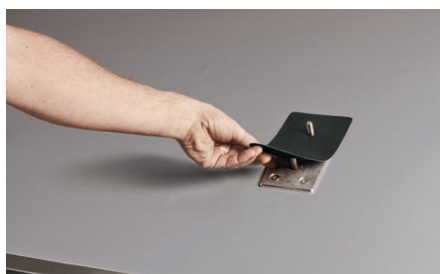
Place larger EPDM intermediate layer
