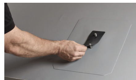
Place smaller EPDM intermediate layer
