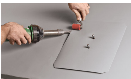
Professional welding of the blank piece
