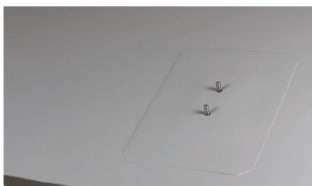
Place larger EPDM intermediate layer
