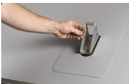
Set Shear-Fix LF 600 over threaded bolt
