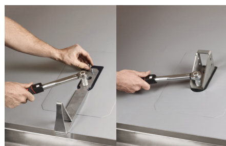
Tighten M10 nuts with 20 Nm to 24 Nm
