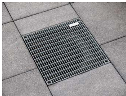
Removable terrace grill with paving slabs.
