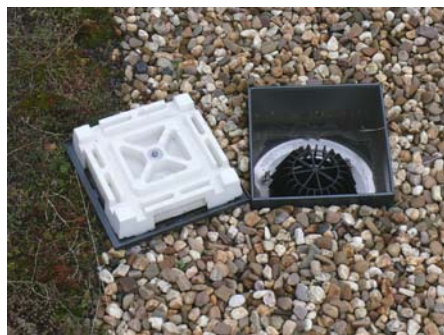
Inspection chamber in extensive green roof.
