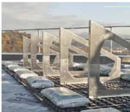
Either a solar energy system or a green roof? That was the past! With the system build-up SolarVert® (Fixodrain® XD 20, ZinCo Solar Base® and basic frame), the combination of solar panels and green roof achieve even greater efficiency. And, there is no need to penetrate the roof membrane as the load required to keep the system permanently stable is provided by the green roof itself. The solar bases can be placed wherever they are required on the Fixodrain® layer.
