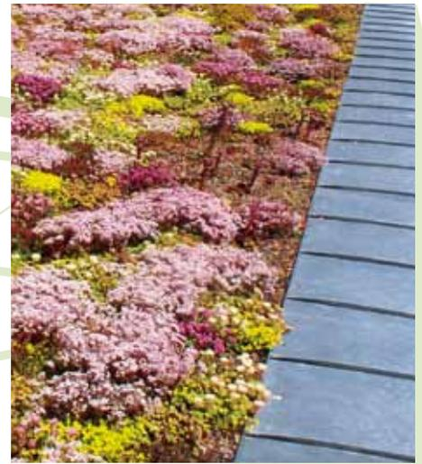
For some roof areas, even the Standard Build-up "Sedum Carpet" is too heavy. The solution is a system build-up with Floraset® FS 75. Less substrate is required as it is not applied equally but mainly fills the gaps between the high studs of the element. Although they start gro-
