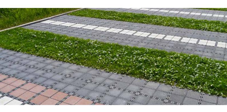
Permeable Ground Reinforcement
